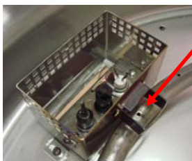
Pilot Window lined up with burner hole.
